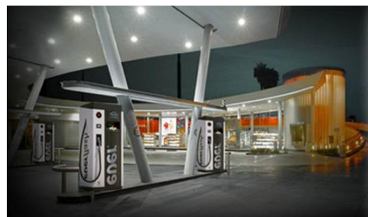
Everflash Charge Station
