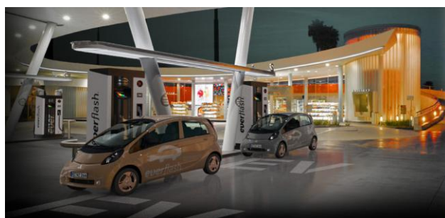
Everflash Charge Station
